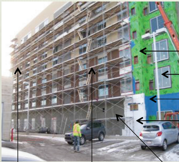
Top Coat Applied Mesh Installed, with Finish Coat Base Coat Applied
