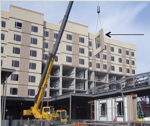
Prefabricated wall panel craned into place.
