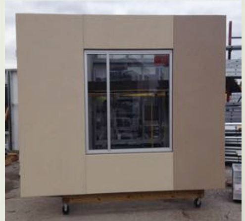
Sheathing Applied Windows Installed Vapor Barrier Applied EPS Foam Installed and Rased
